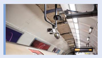
The Arbitex system works with both digital and analogue video systems and provides advanced Al analytic features such as people counting and options to detect specific scenarios to further enhance the safety and efficiency of TfL operations.
